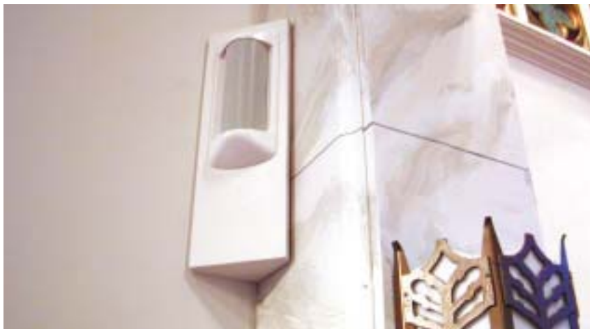
▲ Frank Ward of Acoustical Design Associates chose the TOA H-1 loudspeakers to be unobtrusively mounted and aimed physically close to the seating in this historic 200-year-old landmark chapel.
