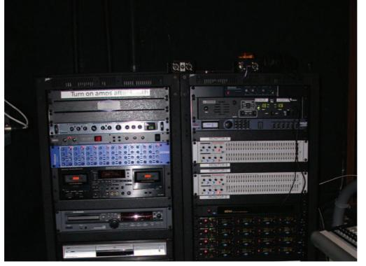
Two Middle Atlantic SR-40-22 racks reside backstage at Clarendon College in Clarendon, TX, and hold most of the sound system's power and effects. The racks were bolted together to move like one piece of equipment, and can be bolted shut for security.
