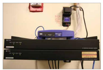
The hands-free intercom system at St. Dominic's Rehabilitation Outpatient Center North is supported by two N-8000EX IP exchange units by TOA Electronics Inc. of South San Francisco. The center is outfitted with 21 master stations located in physical therapy treatment rooms, laboratories, office spaces and by the facility's pool.
